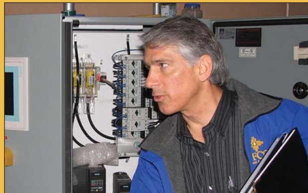
Manager of plant operations Frank Joy gives tours of the woodchip burning boiler, which is expected to save the college $100,000 per year.
